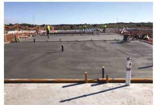
Hatchery construction underway
