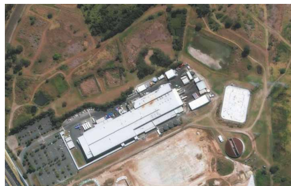
Murarrie site before the pond refurbishment – August 2019
