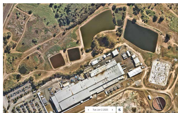
Murarrie site pond refurbishment progress – June 2020
